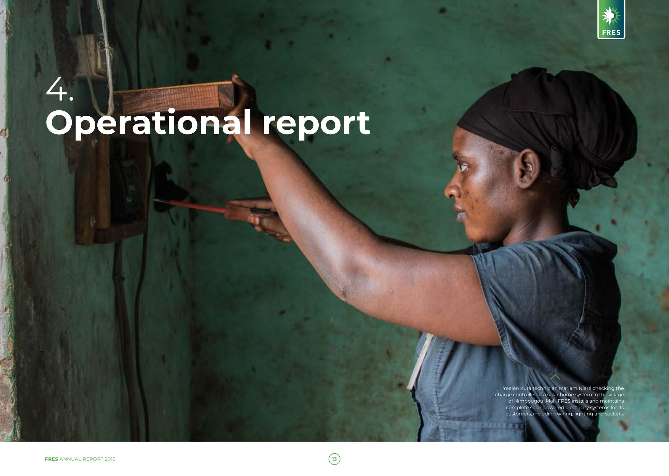
Yeelen Kura technician Mariam Niaré checking the charge controller of a solar home system in the village of Nimbougou, Mali. FRES installs and maintains complete solar-powered electricity systems for its customers, including wiring, lighting and sockets.
