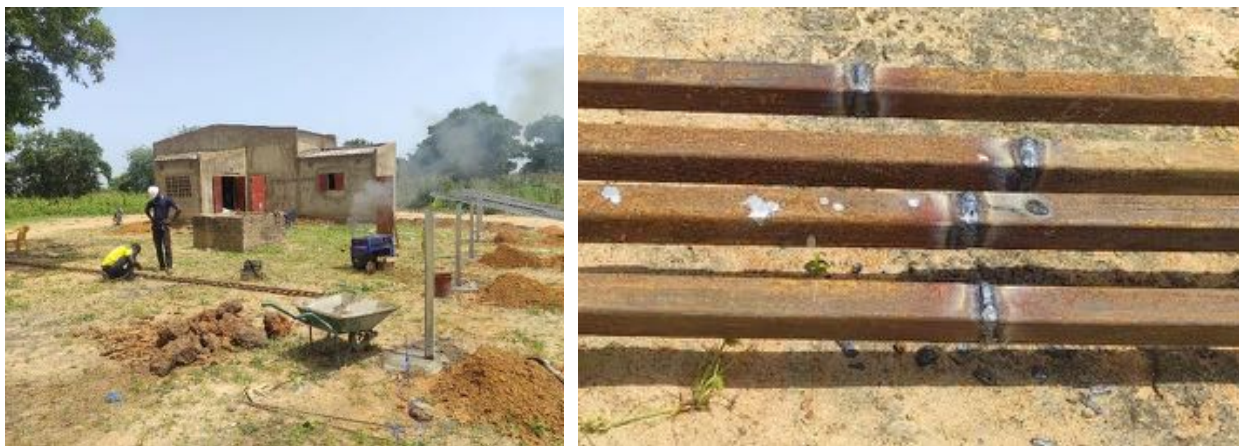
Figure 15 : Drilling the iron tube (crosspieces)
