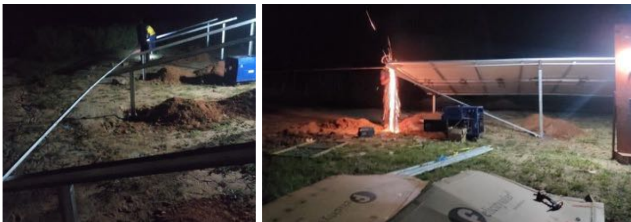
Figure 16 : Soldering the crosspieces
