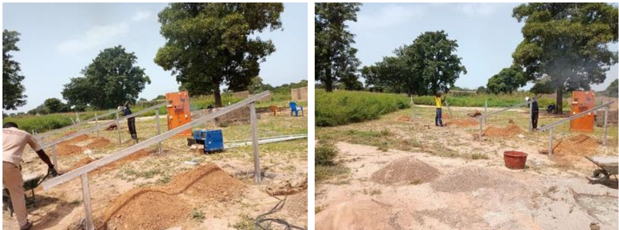
Figure 14 : Soldering the solar panels structures.
