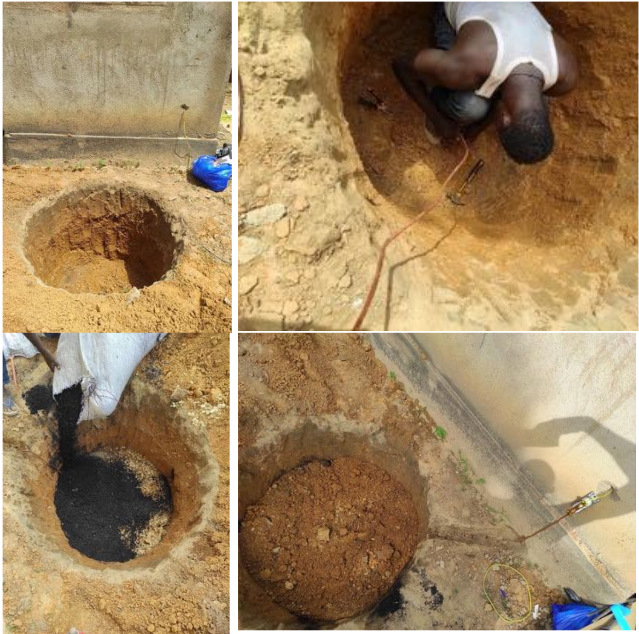
Figure 23 : Grounding steps
