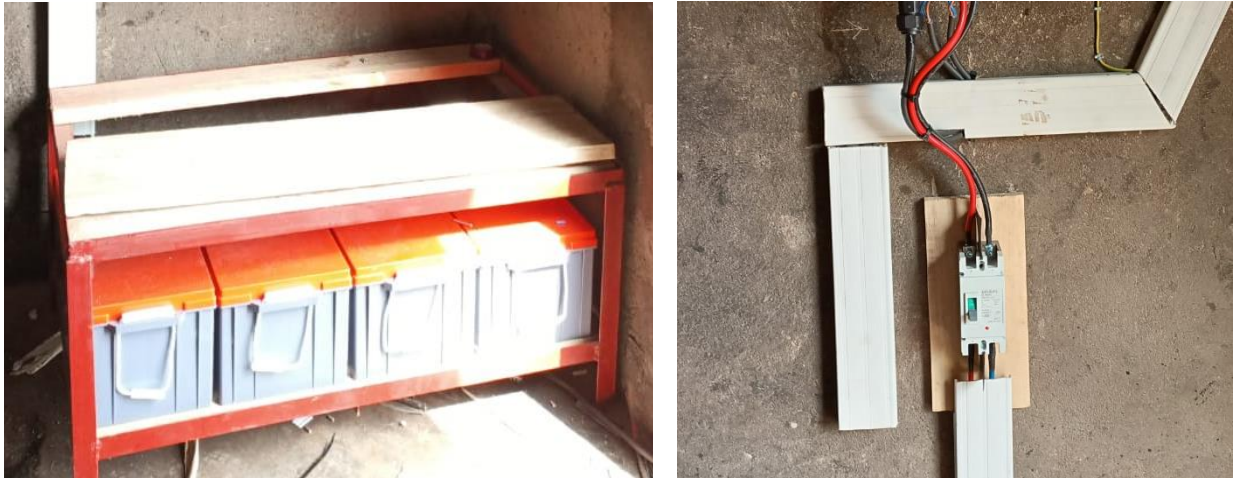
Figure 19 : Batteries plus protection
